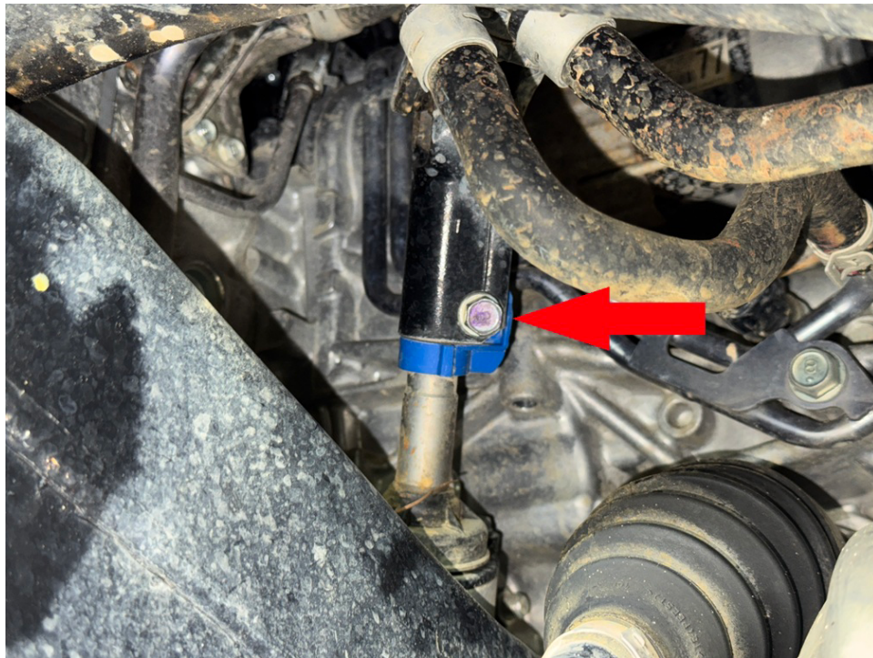
Step 4. Remove bolt holding ground wire to exhaust manifold. Bend mounting tab as shown. Wire will be reattached later.
