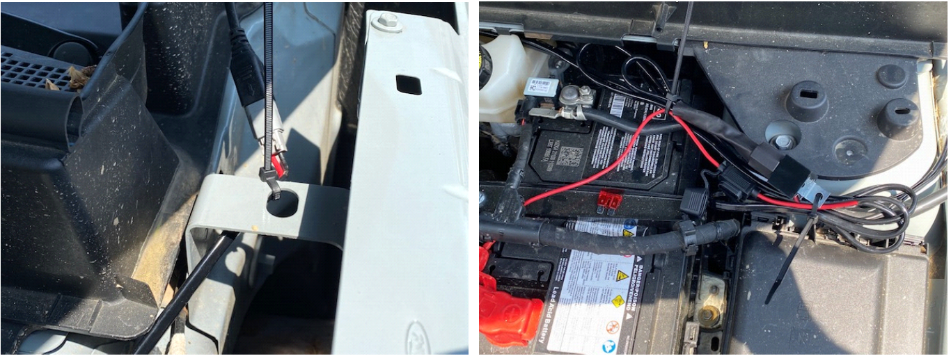
Step 29. Install fuse, test lights.
